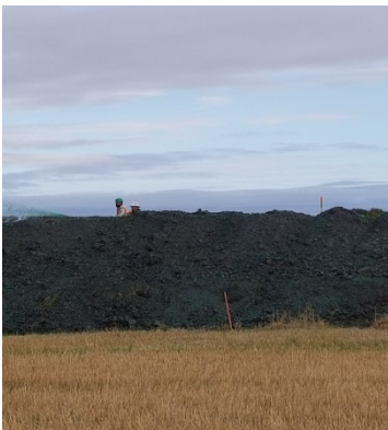
Tackifier at SSKP 1043 area Photo taken facing North
