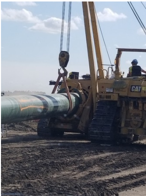
Photo of bending crew at SSKP 045.700 Photo facing South
