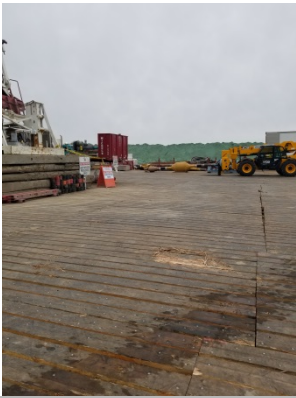
View of some of the HDD site at Dead Horse Creek, photo taken facing North East
