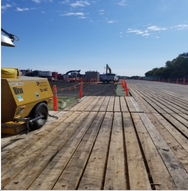
Michel's HDD site at Dead Horse Creek Photo taken facing South
